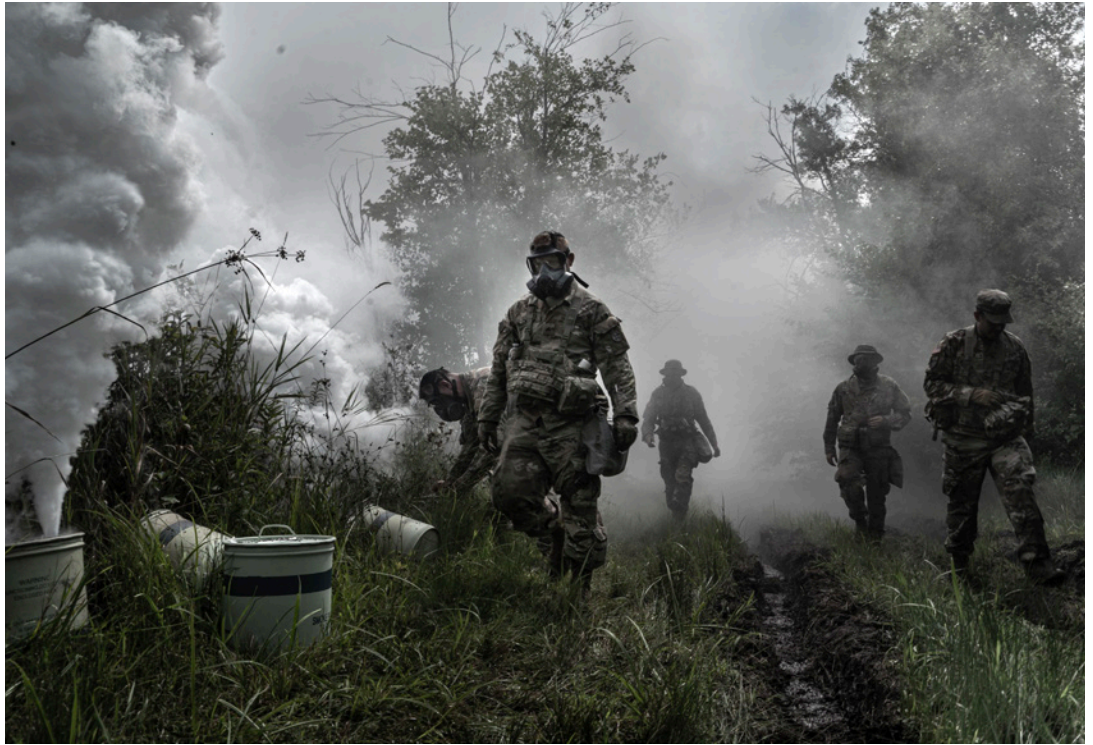
Soldiers from the 351st Ordnance Company provide smoke coverage as engineers construct a multi-role bridge to cross a wet gap at Global Strike 2025 during the Combat Support Training Exercise at Fort McCoy, Wisconsin. (Photo by Staff Sgt. Philip Ribas)
