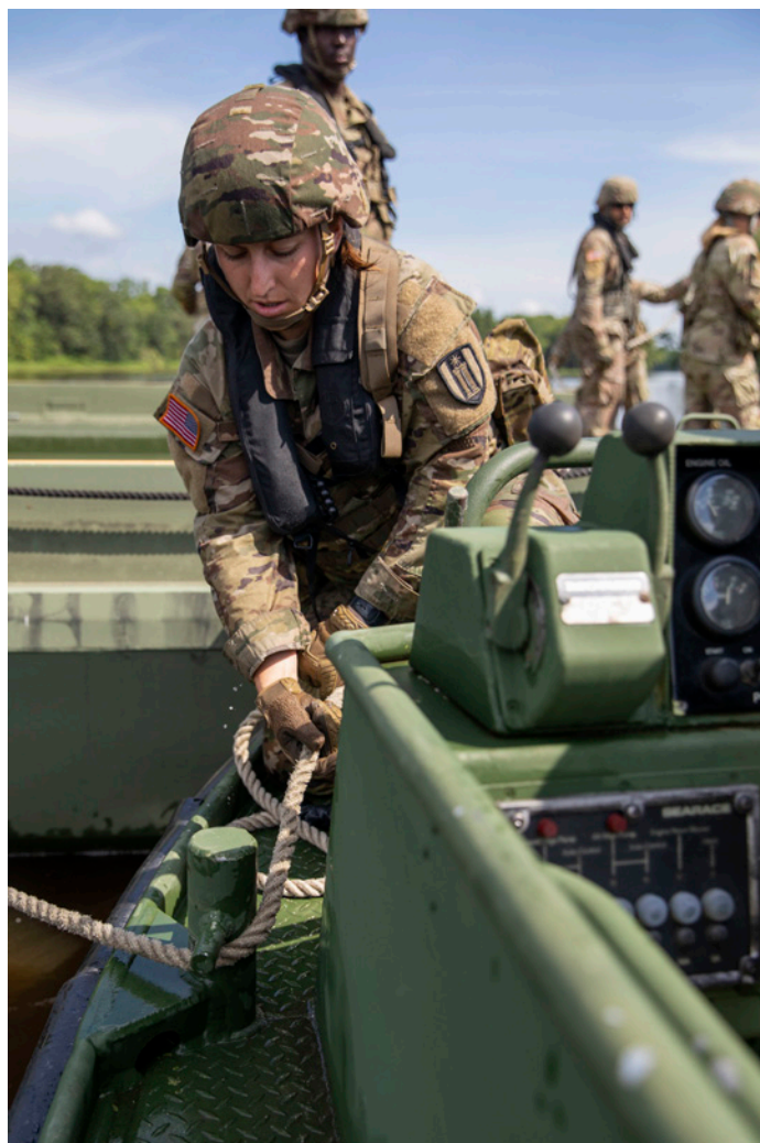
Spc. Ashlyn Jelinek, a bridge builder crewmember with the 652nd Engineer Company, secures a boat to the improved ribbon bridge at Camp Ripley. (Photo by Spc. Elizabeth Hackbarth)
